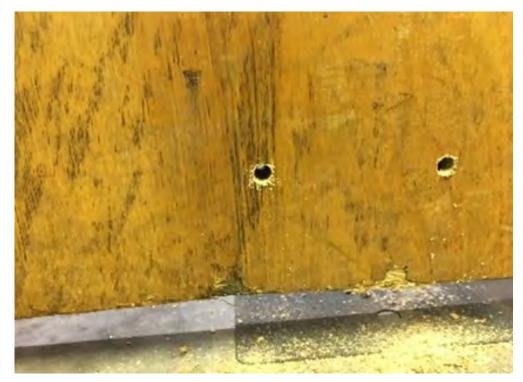
Drill two ¼" holes where the 2 marks are. Be sure to drill straight as this will assure a proper mounting. Drill about half way through from both sides using the 3/8" drill. This will reduce any damage to the door from this process.
