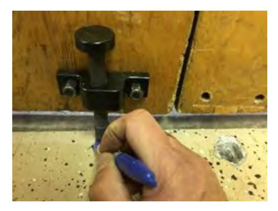
Another way you can mark the floor is you can use a marker and mark around the point where it contacts the floor.
