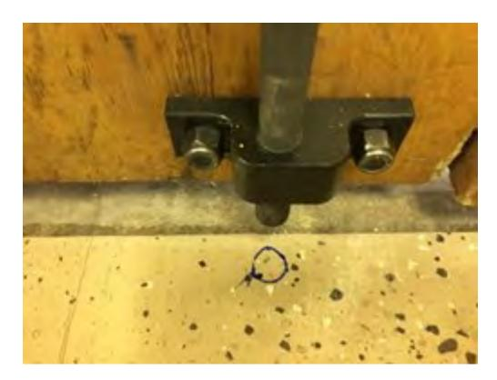
Make sure that the location of the pin is exactly where you want it. For concrete drill in the center of the hole a 1/2" hole using the carbide tipped drill bit and a hammer drill. Then finish drill using the 1" carbide tipped bit. For wooden floors use a 1" wood boring bit.
