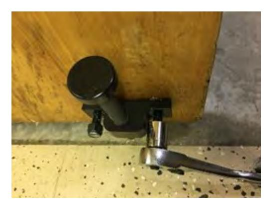
Now slide the Intruder Stop unit onto the bolts and secure with the two locking nuts. (For an install with a threshold, place the spacer block on first then the Intruder Stop unit). Check for square and tighten until the carriage bolts are pulled up tight.
