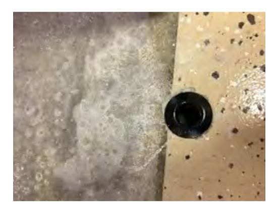
Insert the flanged bushing into the floor.
