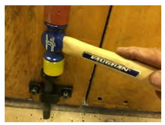
You may now use a hammer and tap the knob down to mark the floor with the built n point
