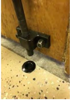
Slide the rod down into the flanged bushing and check for proper alignment. The unit can be adjusted by loosening the mounting bolts and twisting as needed. If the flanged bushing is not correct, open the hole a small amount and reset the bushing and check for fit. The rod should move easily up and down. The rod should stay in place when in the neutral condition.
