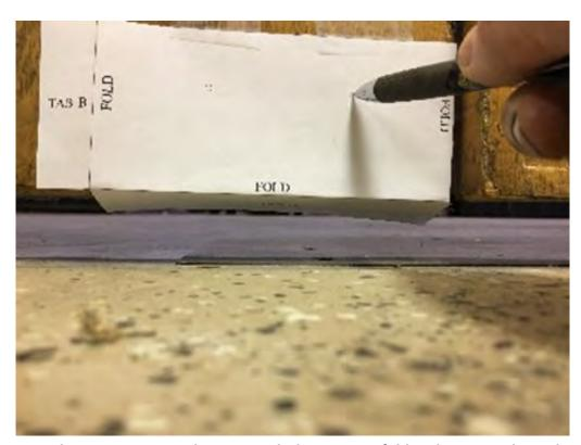
Cut the mounting template out with the scissors, fold on lines as indicated. Tape the template to the bottom and side of the door opposite of the hinges. Using the marker or a sharp punch mark the 2 holes in the template so that a mark is made on the door. This is on the bottom part of the door.
